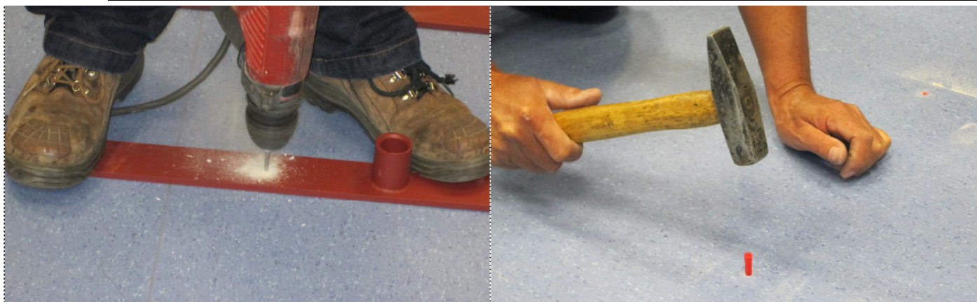
Figure 43: Left: Drill the small holes. Right: Insert plugs in the small holes.
