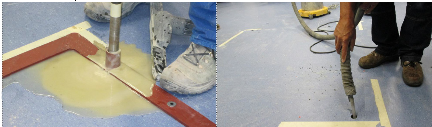
Figure 45: Left: Drilling the hole. Right: Cleaning the holes.
